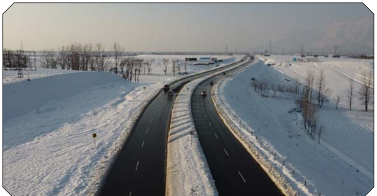
Srinagar Banihal Expressway, Srinagar, Jammu & Kashmir
